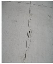
Since drying shrinkage and the resulting tension cracking is totally predictable, both the contractor and the design engineer must prepare for this in both flatwork and walls. The most economical way is to provide control joints which force the unsightly cracks into aesthetically pleasing and maintainable straight lines.
